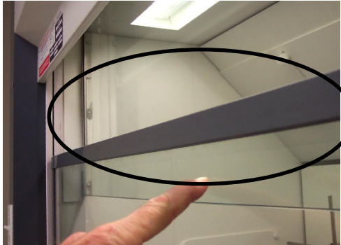
Front-to back overlapping slot bypass
