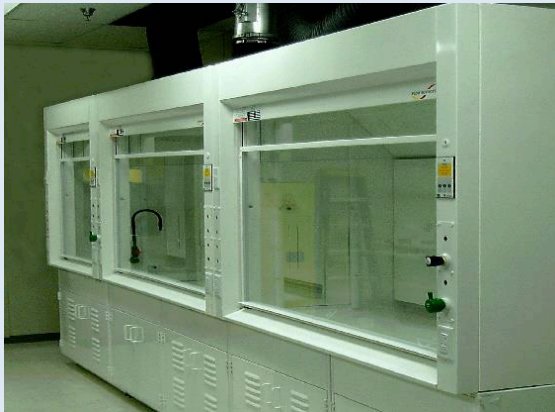
Array of connected fume hoods to handle processes with toxic materials.
